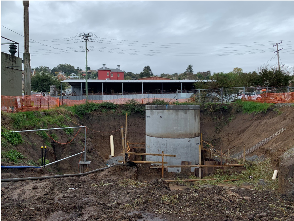
Photo 5: Royal Pump Station wet well installed.
