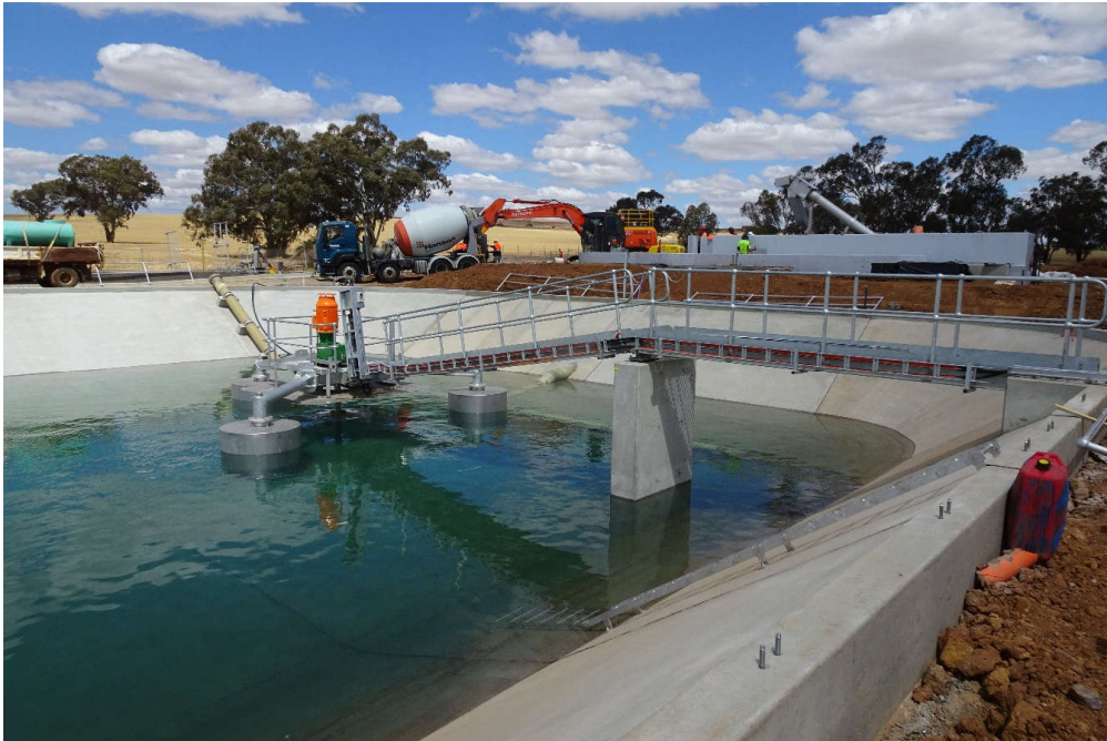
Floating Surface Aerator on bridge (Sewage Treatment Plant at Junee Shire Council)
