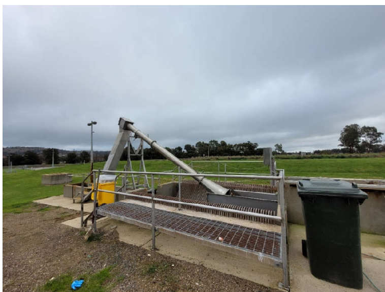
Figure 4 - Inlet Works at Cootamundra STP
