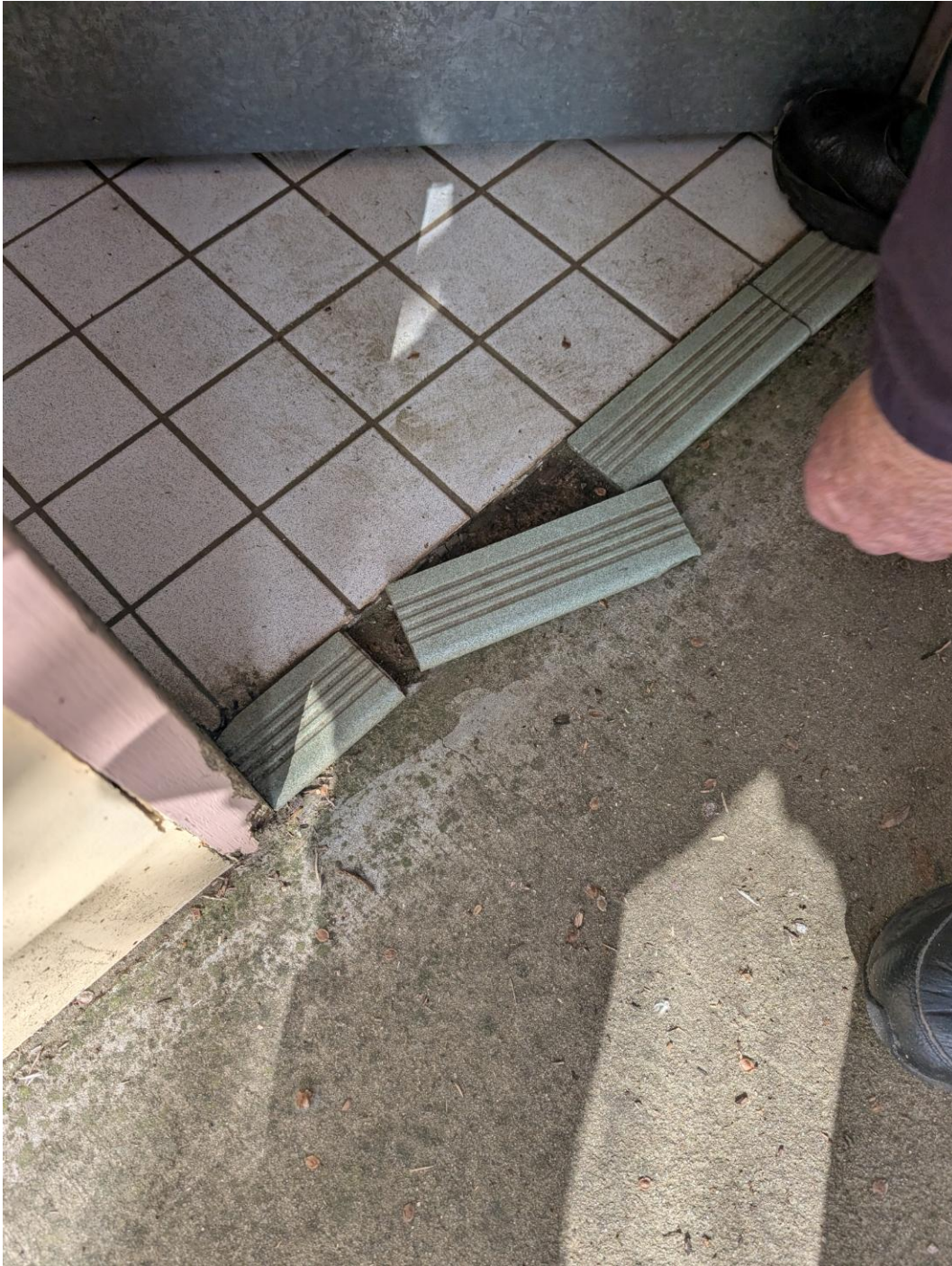
Location: Entry door to female toilets
