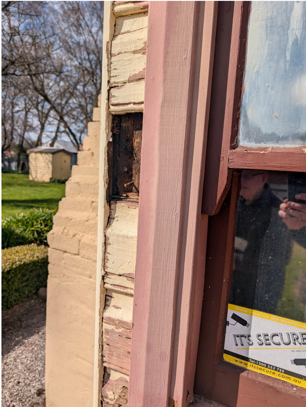
Location: Rear entry door to Bradman Museum cottage
