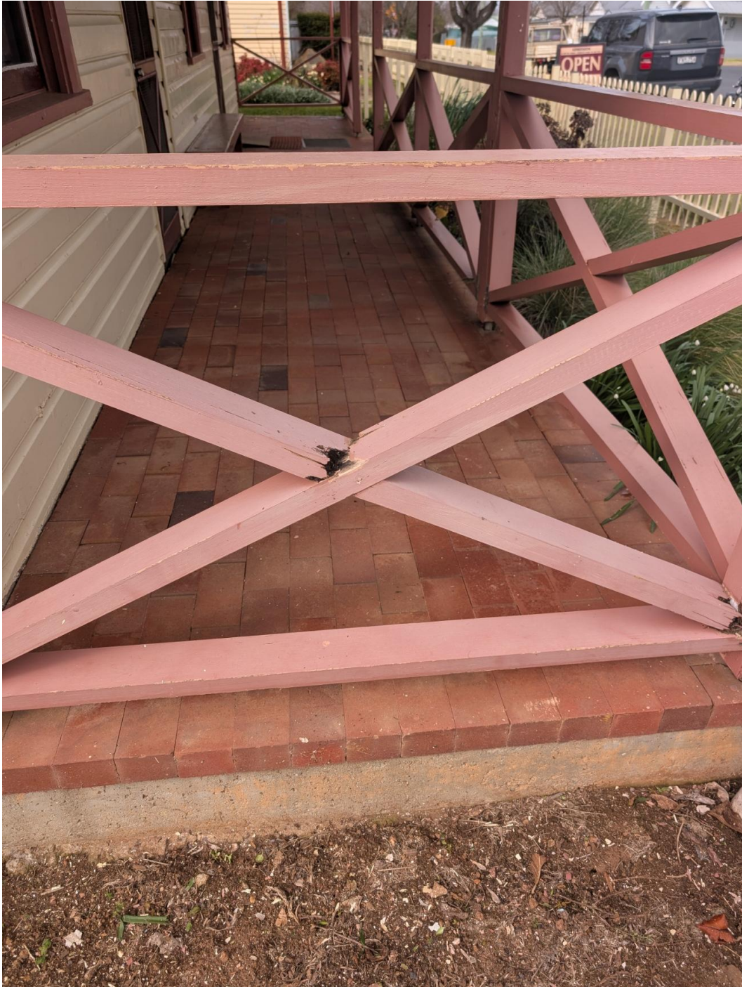
Location: Verandah, adjacent to main entry door to Bradman Museum cottage
