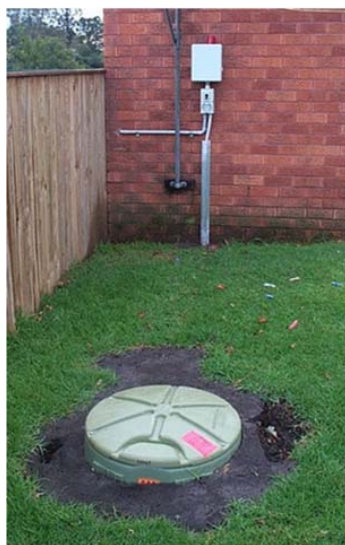
Figure 3-3: Typical Installed Pressure Unit
