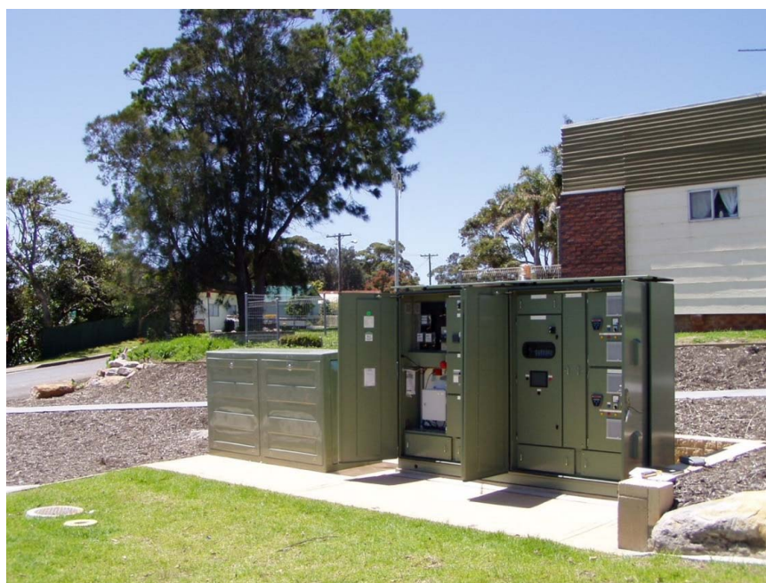
Figure 3-13: Typical SCA Installation
