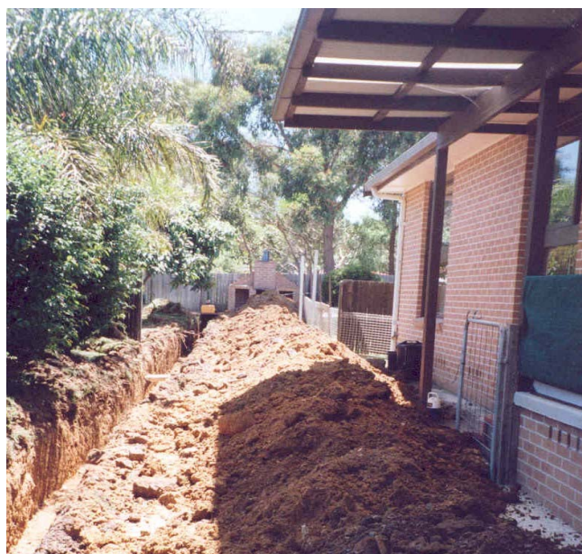
Figure 3-11: Installation of Gravity Pipeline in a Back Yard
