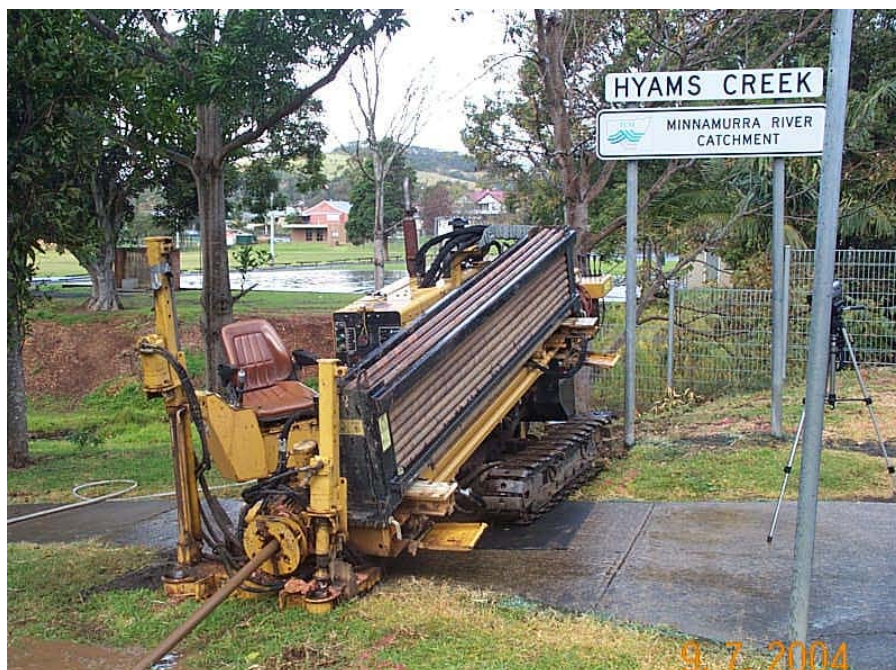
Figure 3-8: Directional Drilling Equipment for Pressure Sewers
