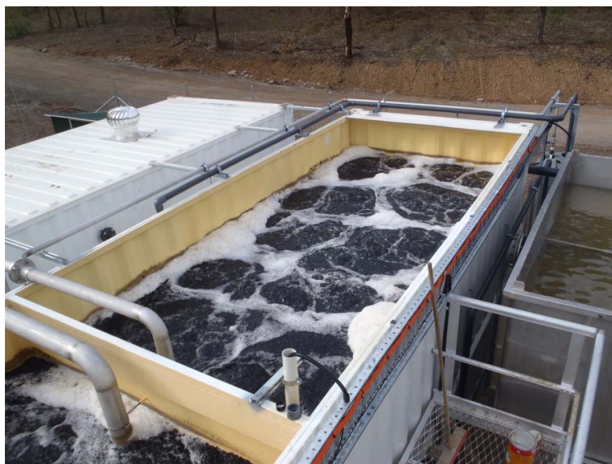
Figure 4-5: John Morony STP – Package Treatment System
