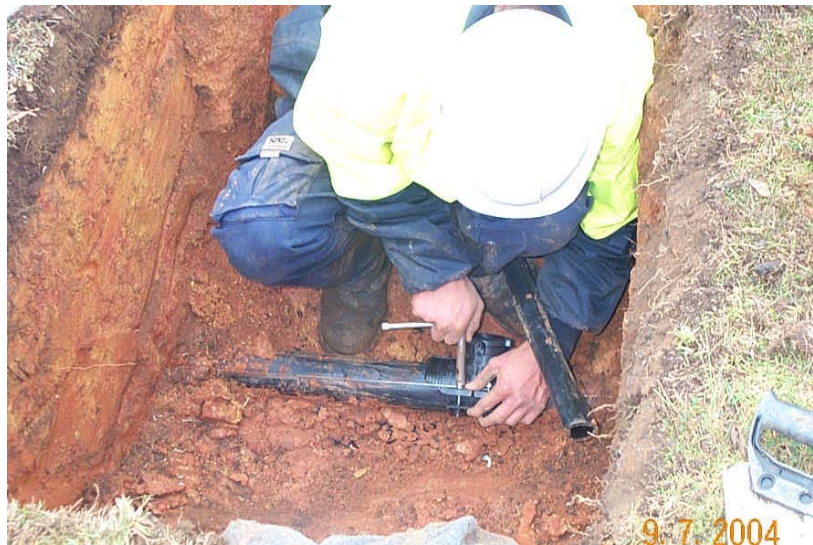
Figure 3-6: Completion of Pipe Connections
