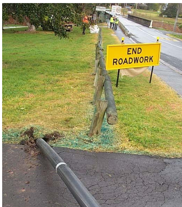
Figure 3-9: Pipelaying in Progress via Directional Drilling
