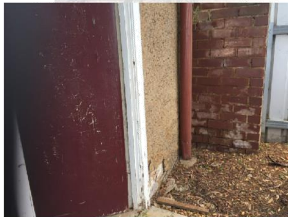
Gutter water overflow outside Kitchen
