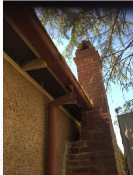
"Hanging gardens" and grass growing in rusted gutter
