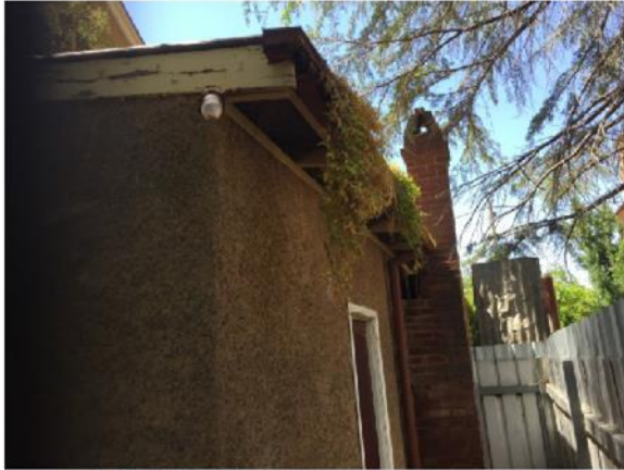
"Hanging gardens" and grass growing in rusted gutter
