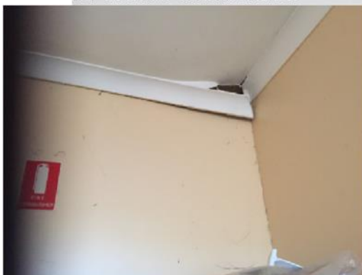
Gutter water overflow outside Kitchen
