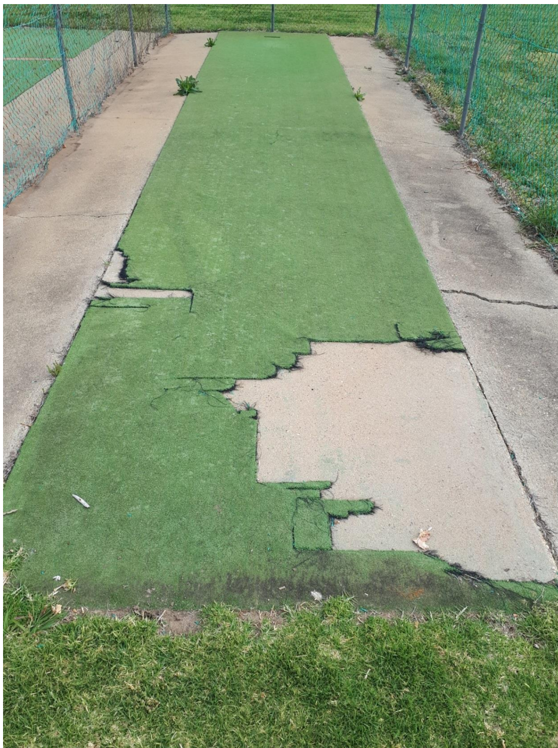
Figure 8 - The existing synthetic grass has aged and now creates too much bounce for the cricket ball. Not only can this be dangerous to the batsman it also fails to provide the kids genuine cricket training as the wickets they play their games on bounce much lower.
