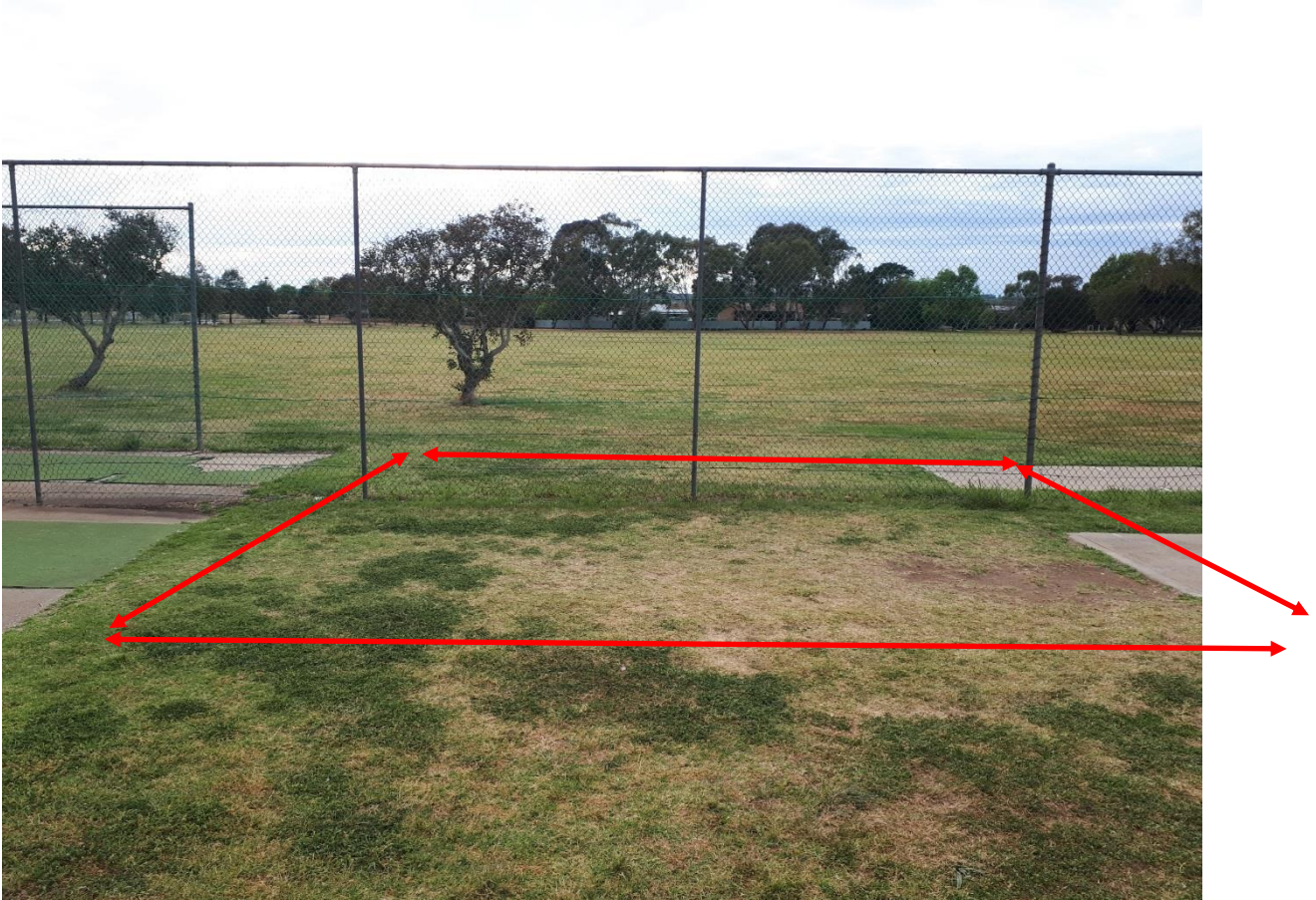
Figure 2- The grass between the two concrete slabs need to be removed and concreted.
