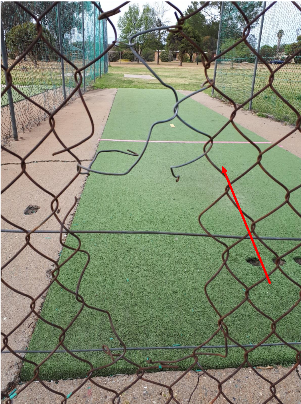
Figure 1- Hole in existing net
