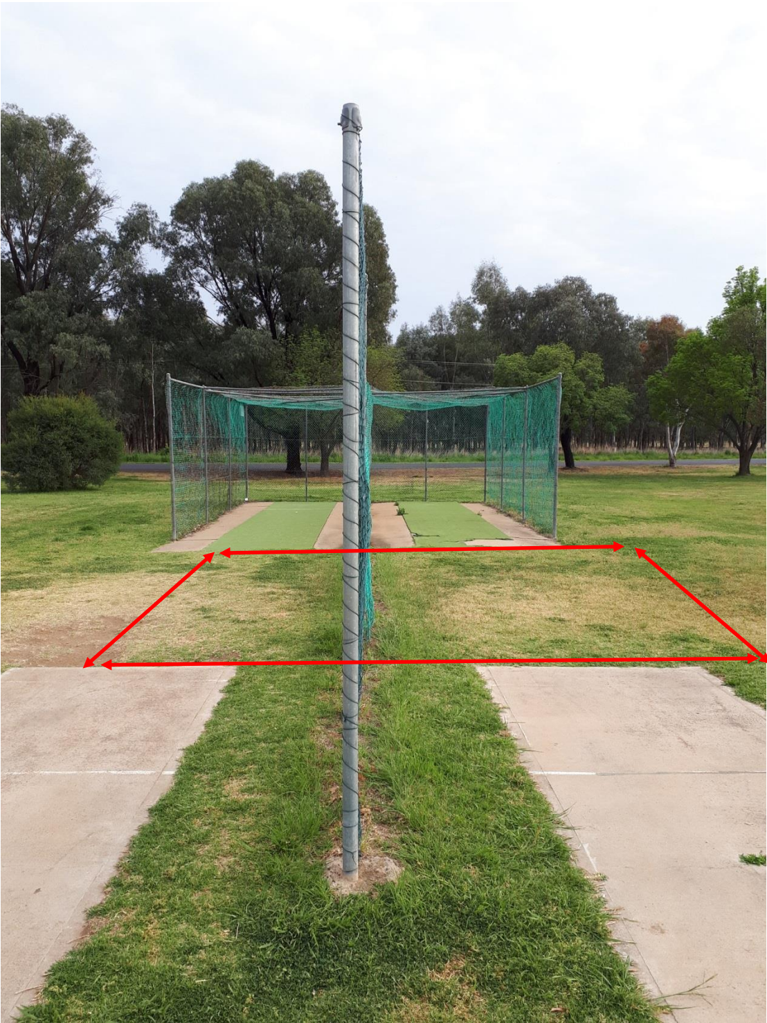
Figure 3- The grass between the two concrete slabs need to be removed and concreted.
