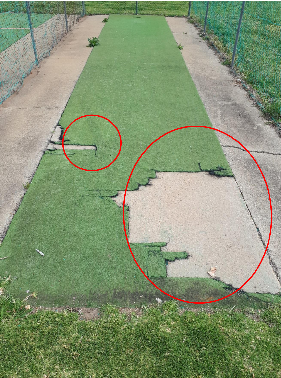
Figure 5- The synthetic grass on one of the wickets is severely damaged.
