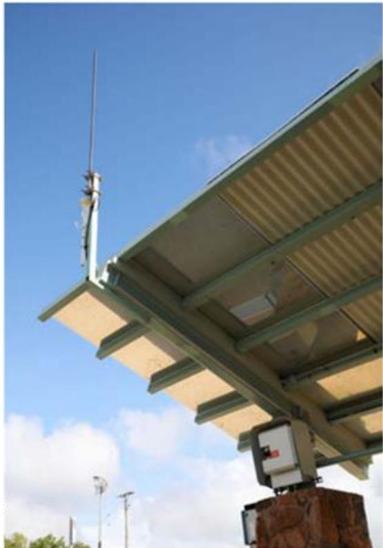
Taggle's Byron network is comprised of base stations that include extremely sensitive radio receivers fitted with a high gain antenna.
