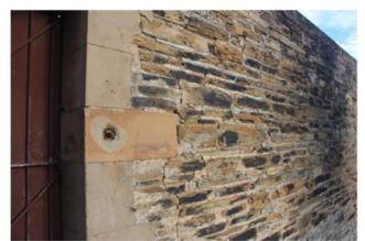
Figure 13: The walls enclosing the old gaol complex feature local slate
