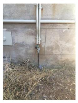
Figure 8 - Cell Block Earth Stake
