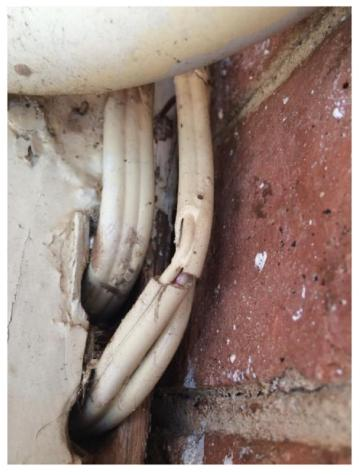
$\textit{Figure 35-Infirmary Block Recent Electrical Installation Damage \textit{(External)}}\\$
