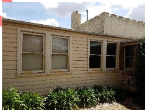
Plate 225. Weatherboard extension to the rear of the house. Some deterioration of paint around windows and on the weatherboard.
