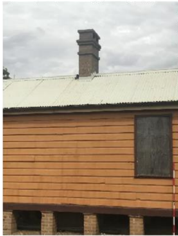
Plate 194. Brick chimney in the centre of the galvanised pitched roof.
