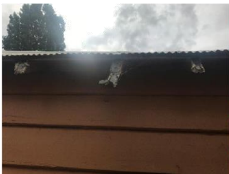
Plate 200. Damage to roof and guttering
