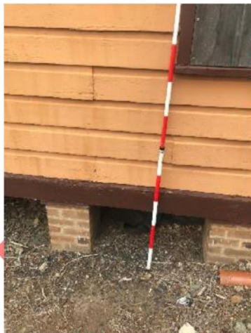
Plate 196. Weatherboard structure on brick stilts.
