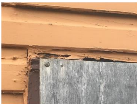
Plate 204. Damage and peeling paint above the boarded-up doors and windows.
