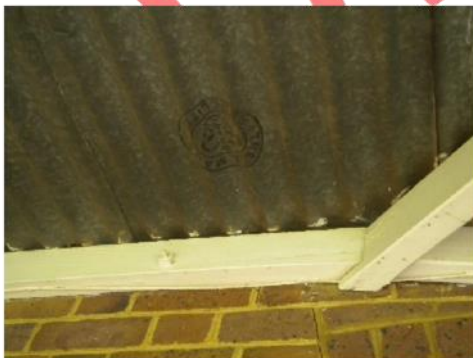
Plate 39. Galvanised roof with Trade mark symbol
