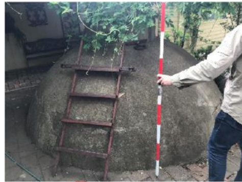
Plate 245. Well covered with a concrete dome.
