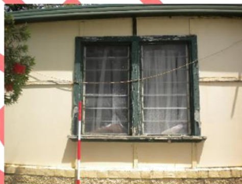
Plate 62. Significant paint degradation on window frame.
