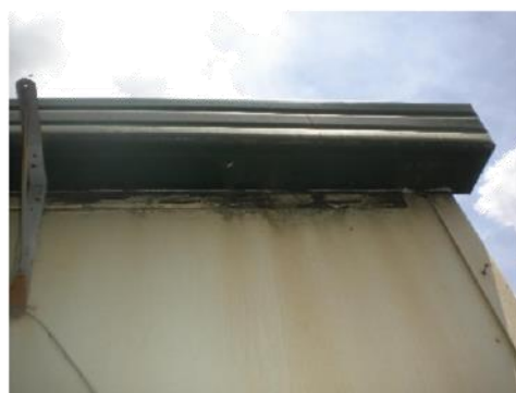
Plate 64. Mould and Mildew growth underneath the eaves of the building.
