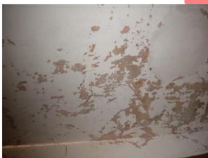
Plate 180. Paint peel and deterioration.
