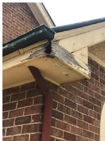
Plate 107. Significant deterioration of the guttering on the southern façade of the Church. A hole has worn through the wooden material.
