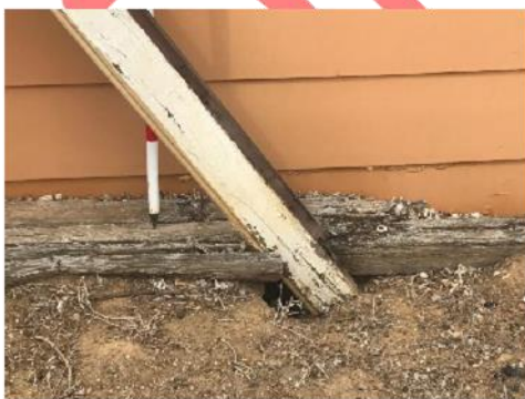
Plate 202. Damage and rot to wooden beam that has fallen off the guttering on the roof.
