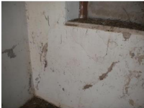
Plate 174. Significant paint deterioration and peel.
