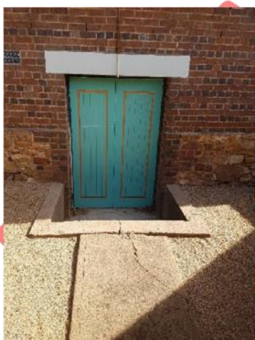
Plate 131. Access door set down into the wall accessed by cement stairs.
