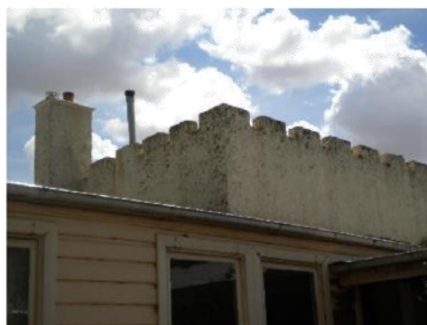
Plate 237. Mould and mildew growth on the upper sections of the battlements.
