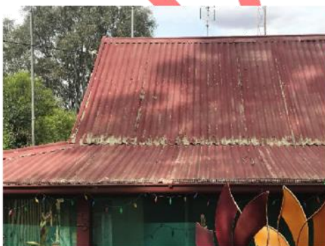
Plate 242. Faded galvanised roof with steep pitch.
