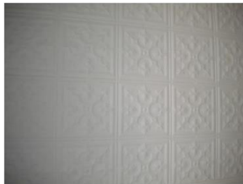
Plate 40. Pressed metal roof.
