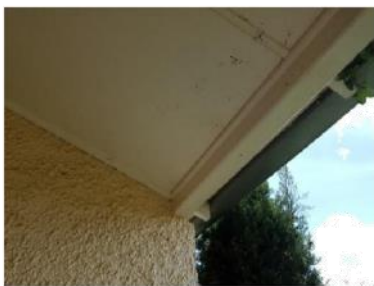
Plate 220. Verandah ceiling with mould growth and inhabited by invertebrates.
