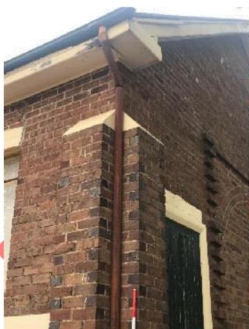
Plate 104. Corner detail of the church. Note the deteriorated paint on the guttering and doorway.
