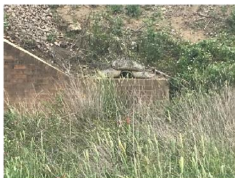
Plate 211. Brick wall of Railway Underbridge with pipe covered by sandbags.
