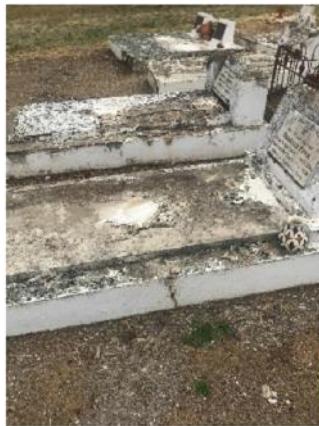
Plate 21. Mould and mildew build up on numerous grave stones.
