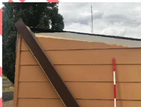
Plate 201. Damage to roof with the guttering pulling away from some areas.
