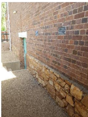
Plate 129. Northern façade (rear) of building. Brick work over stone. Access door set down into the wall accessed by cement stairs.
