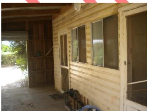
Plate 236. Some deterioration of paint on the weatherboard.
