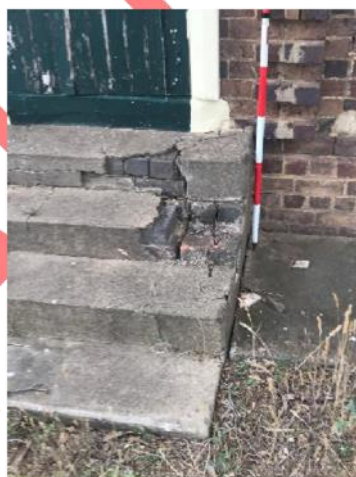
Plate 101. Significant damage to rendered bricks used to enter and exit the back door of the church.
