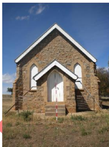
Plate 159. Southern (front) Façade of former Presbyterian Church. The building is constructed in locally sourced granite stone with a galvanised roof.
