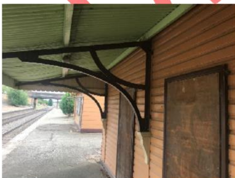
Plate 192. Metal brackets supporting roof.
