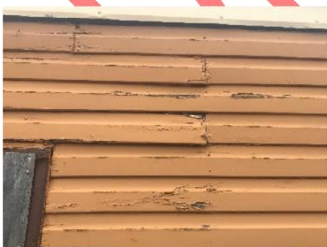
Plate 186. Damage and paint rot to the weatherboard building.
