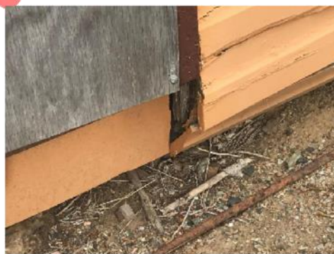
Plate 203. Damage and rot to the wood join.
