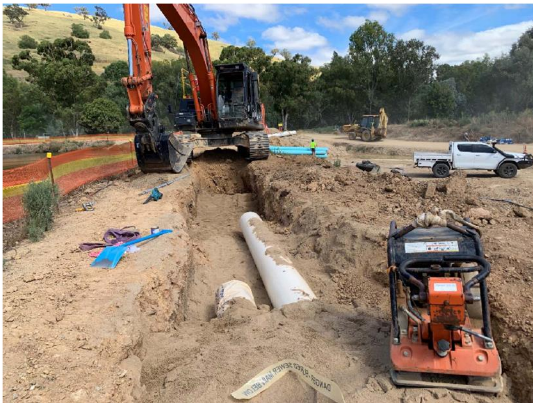
Photo 5: Construction of effluent outfall pipeline in progress.
