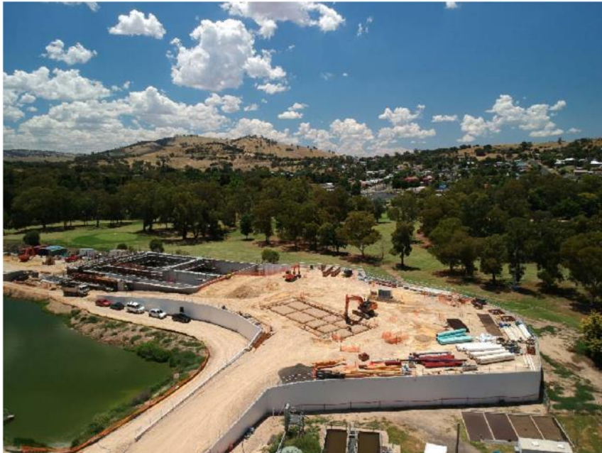
Photo 1: Gundagai STP site, aerial view looking North.
