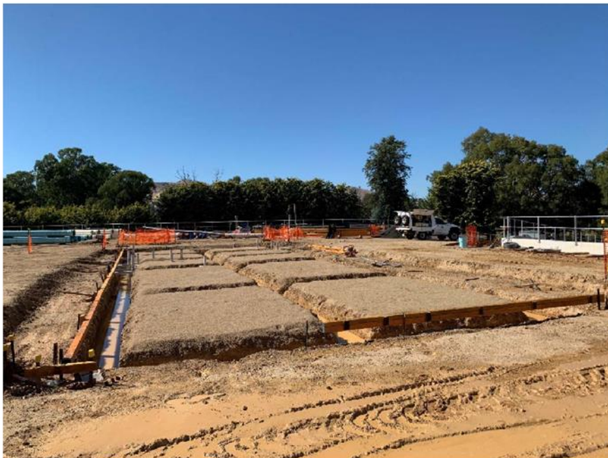
Photo 4: Foundation preparation for amenities building.
